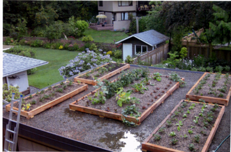
Green roof off and running. The finished rooftop vegetable garden is watered using rain collected from rain barrels.
