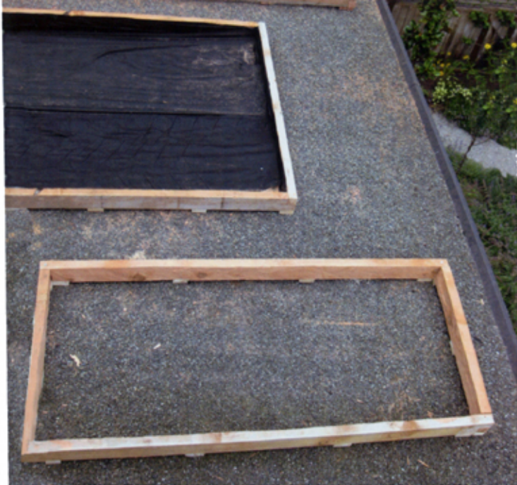
Building boxes. Gravel on the roof provides positive drainage
